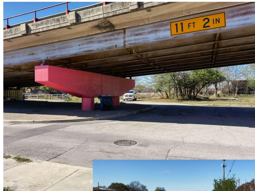
MH #38159 – Under Guadalupe St. Bridge
