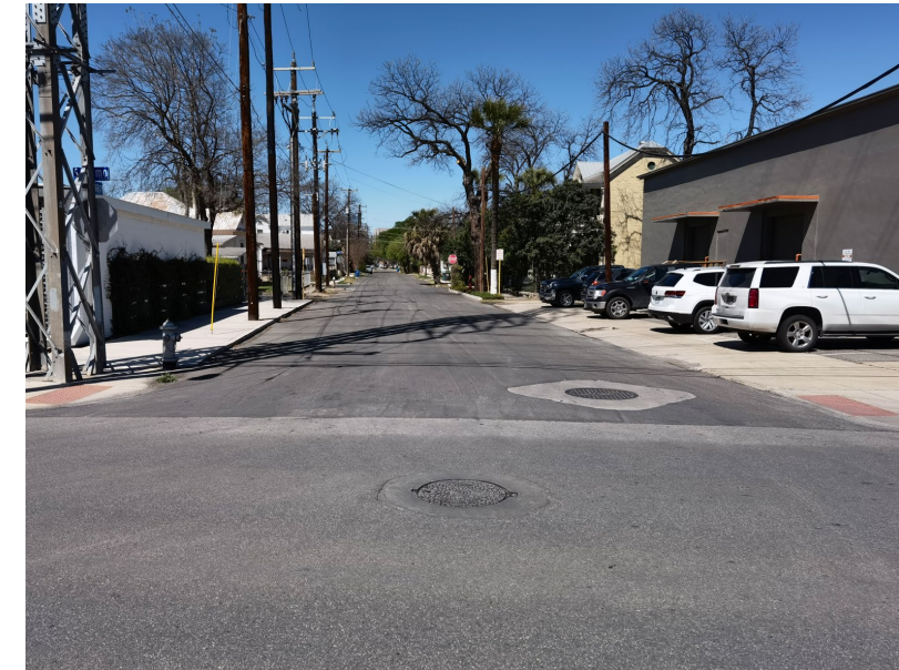
MH #25672 – Looking North on Nathan St.
