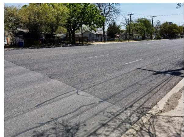
Facing south down Zarzamora St towards W Harlan Ave
