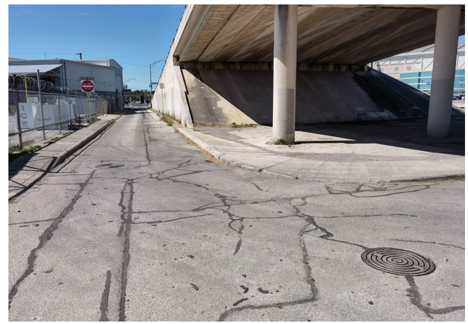
MH #27141 – Looking NW under E Cesar Chavez Blvd Bridge
