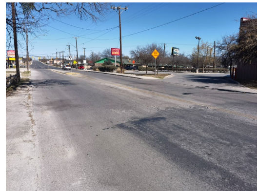
Facing west down Roland Ave
